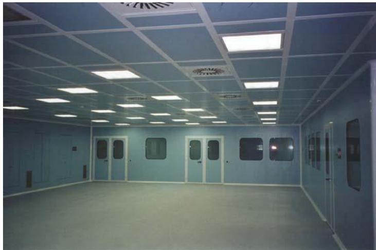
The thickness of the **CT-CLEANROOMS** panels is 48 mm; this thickness permits the integration of enclosed electrical arrangements for switches and sockets, optical indicators for doors status, coplanar return air grilles and inspection removable panels for the passage of utilities.
